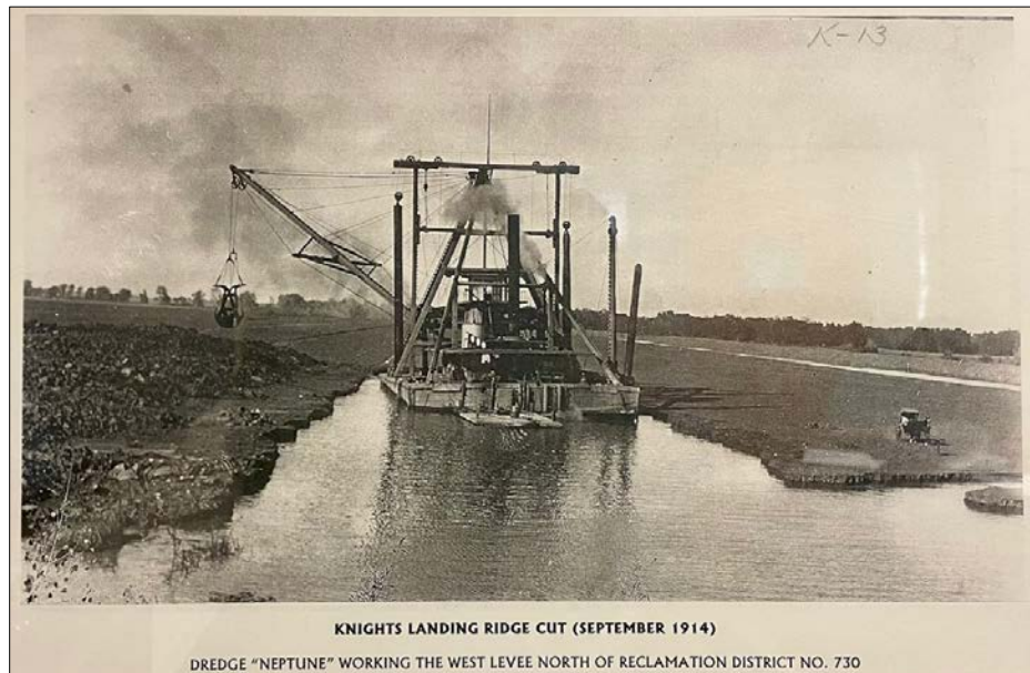
DREDGE "NEPTUNE" WORKING THE WEST LEVEE NORTH OF RECLAMATION DISTRICT NO. 730
