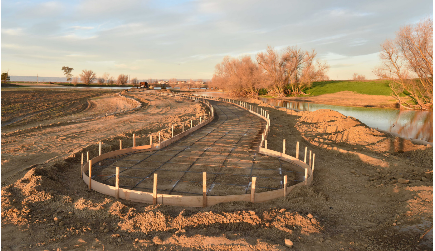
Woodland Regional Park Trail project construction. Photo Credit: Lars Anderson
